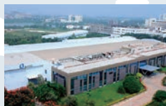
Bangalore Plant 59,000m 2
