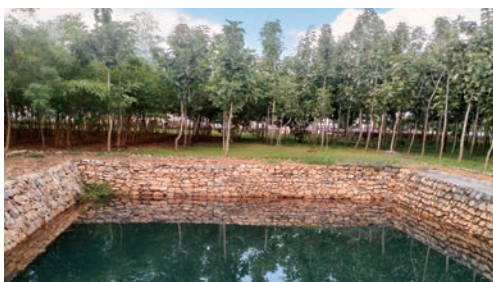
Reservoir at Coimbatore Plant
