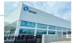
Wuhan Plant 174,000m 2
