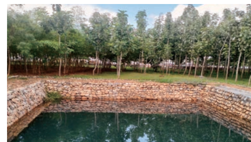
Reservoir at Coimbatore Plant
